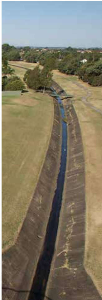
The existing concrete storm water channel.
